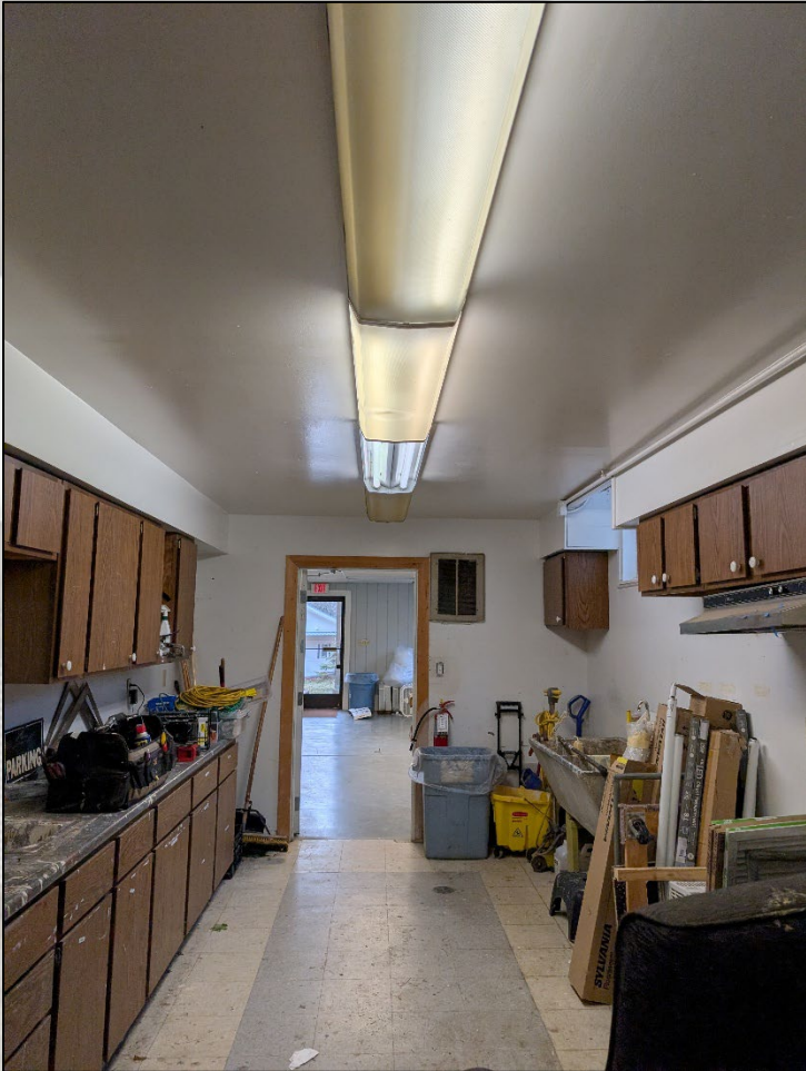
Maintenance Room – (6) 60w T12 bulbs to (6) LED 25w T8 bulbs 360w >> 150w total
