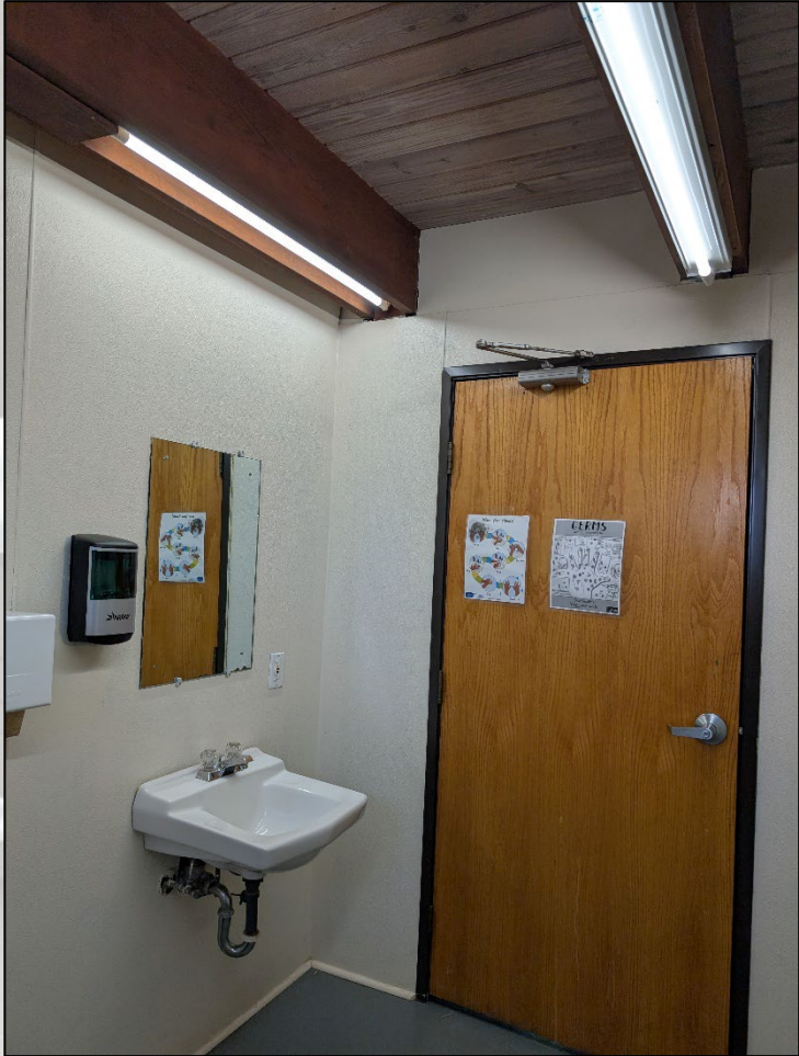
Maintenance Room – (6) 60w T12 bulbs to (6) LED 25w T8 bulbs 360w >> 150w total
