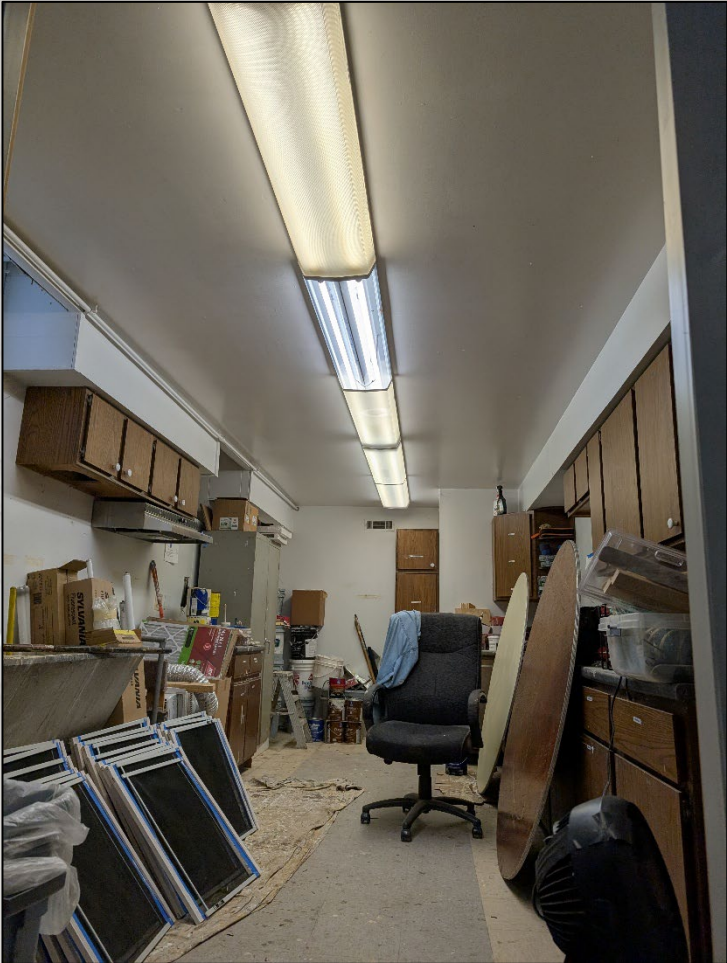
Maintenance Room – (6) 60w T12 bulbs to (6) LED 25w T8 bulbs 360w >> 150w total
